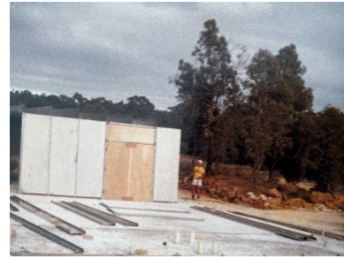
First wall up!
