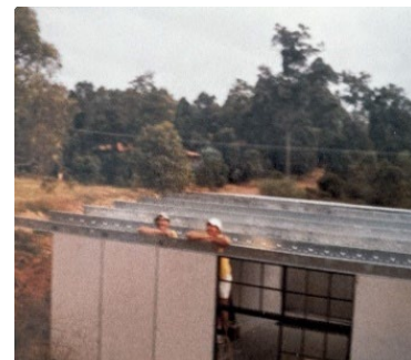
No roof yet! Don Burgess, Derek Townsend
