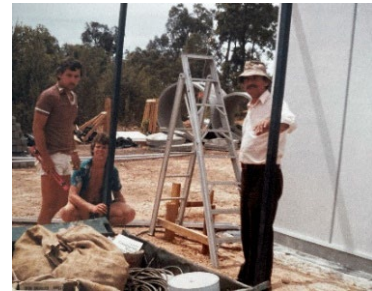
Second wall about to go up!
